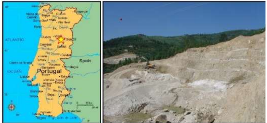
Figure 1. The location of Alvarrões lepidolite mine, Portugal. (Source: Company).
