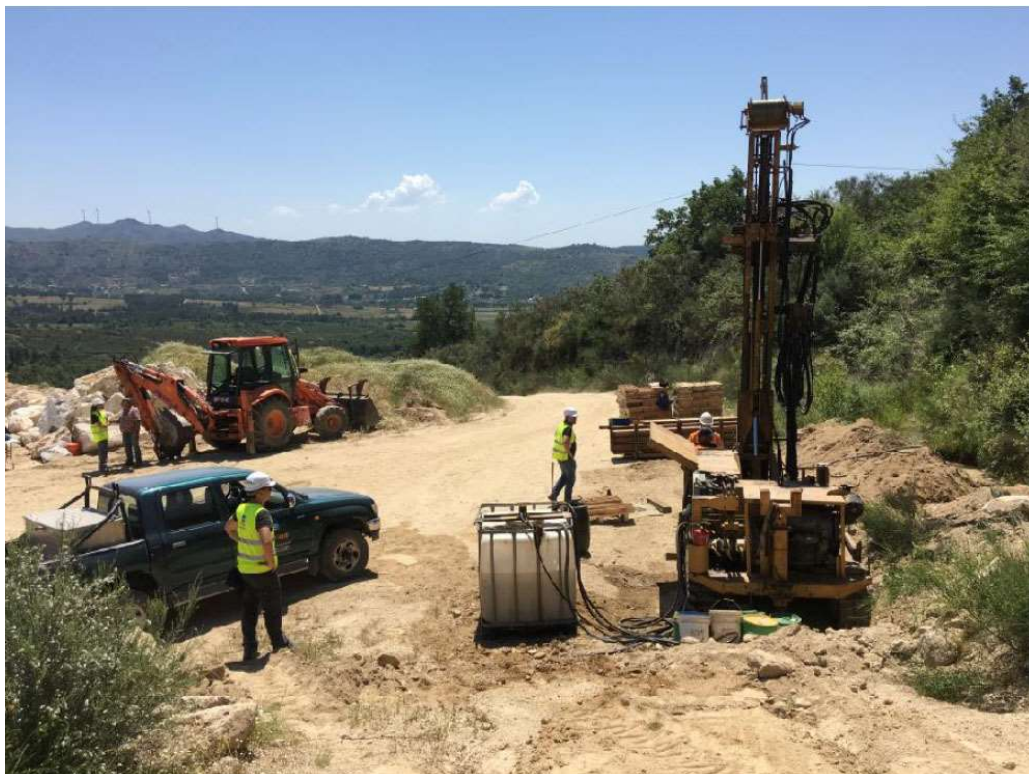
Figure 4. Rig set up on the first drill hole at Alvarrões lepidolite mine, Portugal. (Source: Company).
